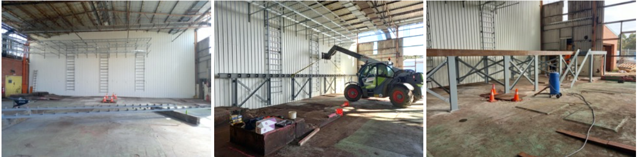
Above: (left) cable trays in place, ready to commence MCC construction, (centre & right) MCC floor construction.
