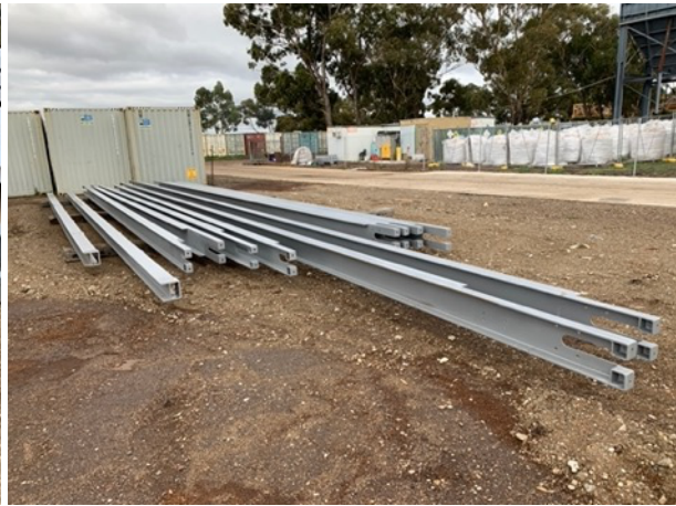
Above: vertical structural supports (left) & conditioning belt horizontal structural supports (right).
