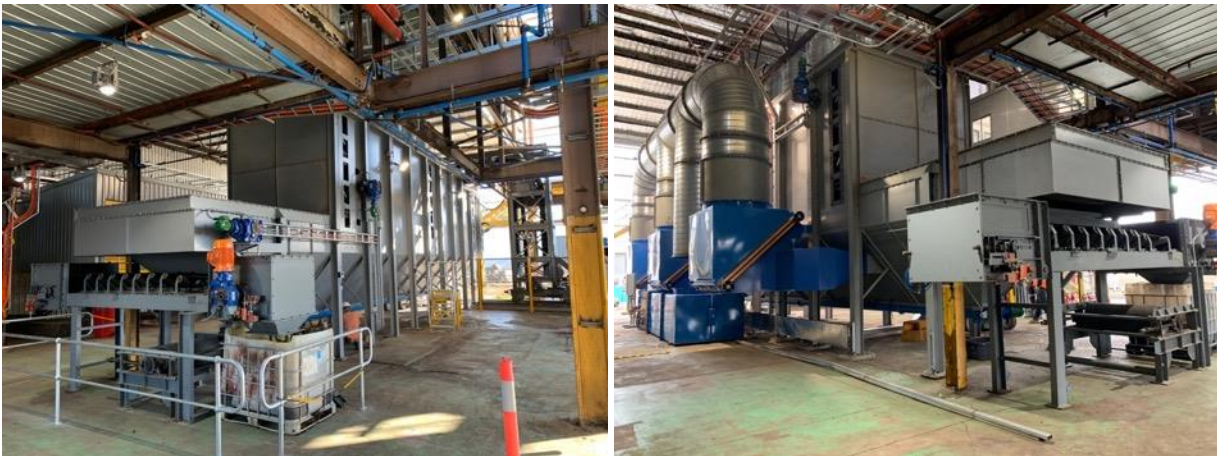
Photos (above): conditioning system commissioning.
