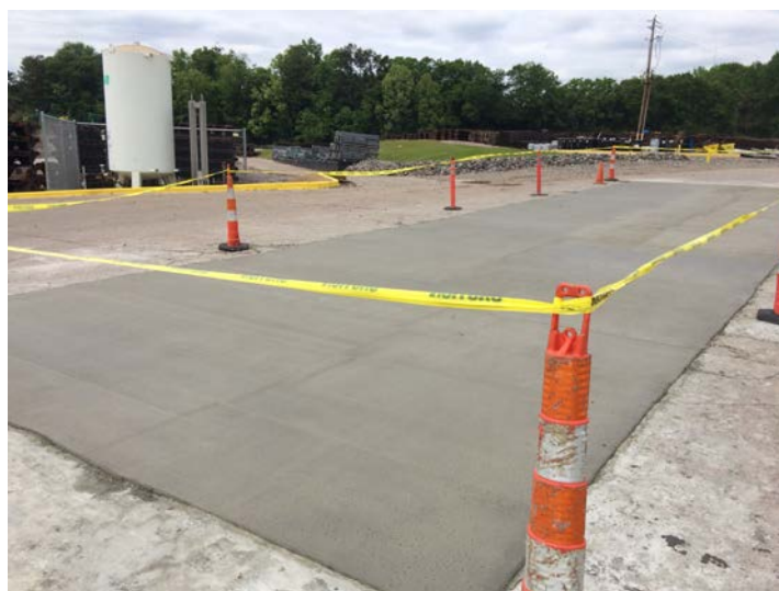
Figure 6. Completed first slab
