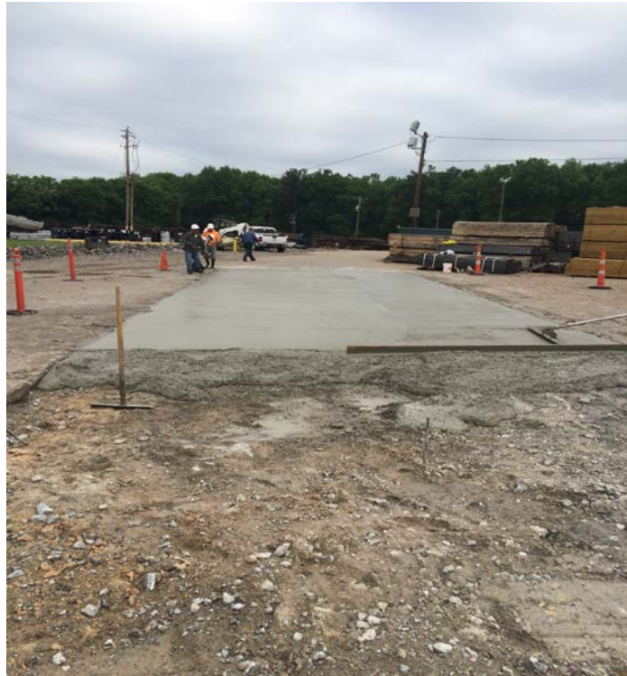
Figure 5. Partially poured first slab showing minimal sub-base preparation
