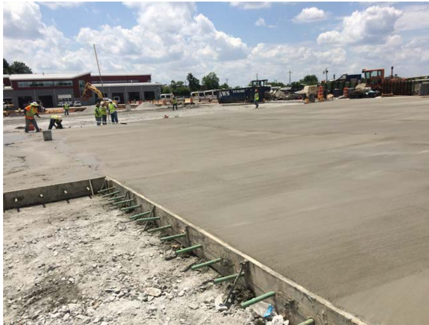
Figure 2. EdenCrete™ enriched slab being installed
