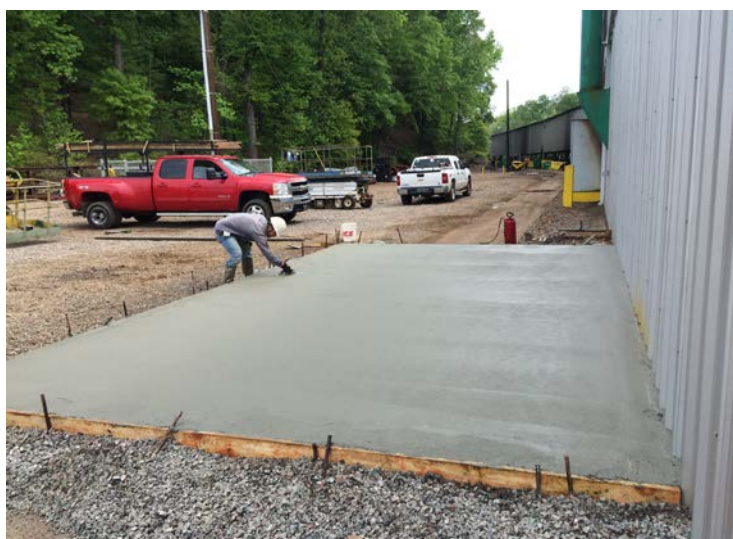
Figure 8. Completed second slab
