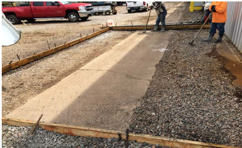
Figure 7. Formwork and minimal sub-base preparation for second slab
