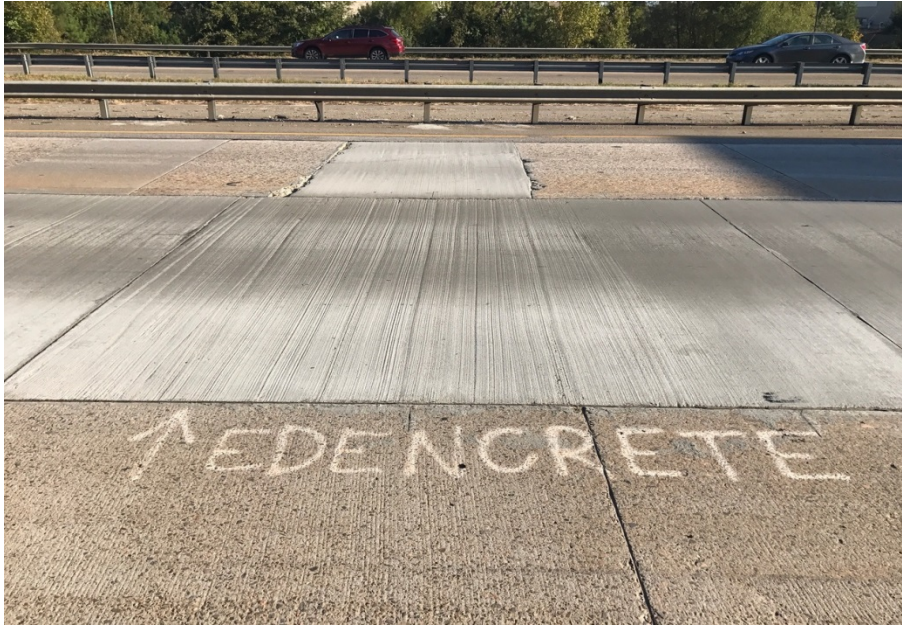
EdenCrete™ – No Visible Cracking
