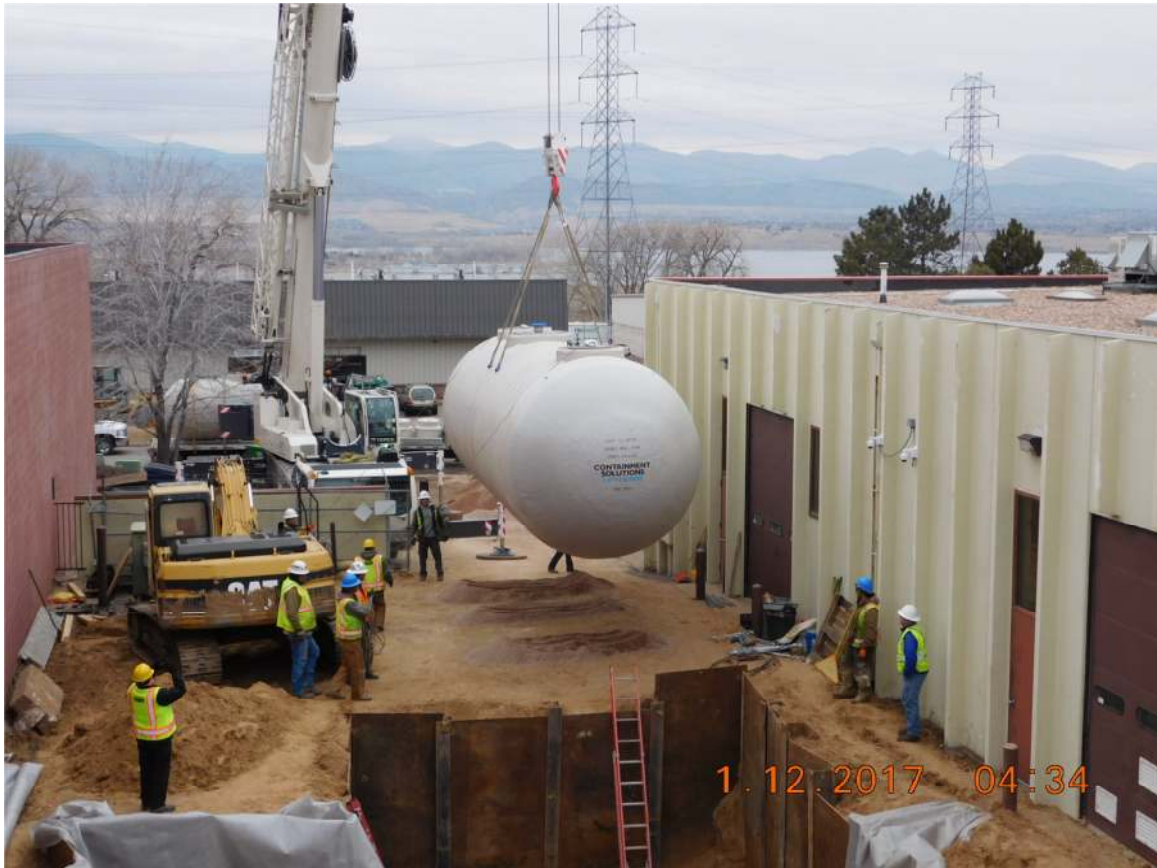
Figure 1. One 20,000 gallons capacity EdenCrete™ underground storage tank being installed
