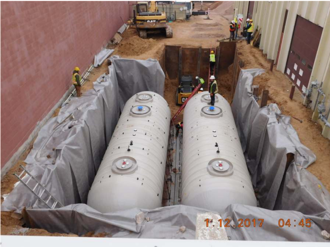
Figure 2. Two 20,000 gallons capacity EdenCrete™ underground storage tanks in place
