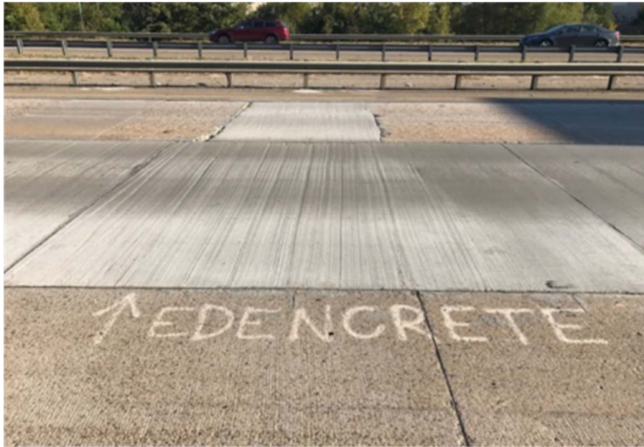
EdenCrete® – No Visible Cracking
