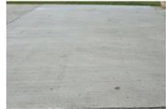
EdenCrete Trial Slab No cracks or evidence of wear
