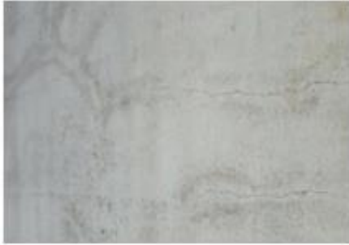
Control Trial Slab
