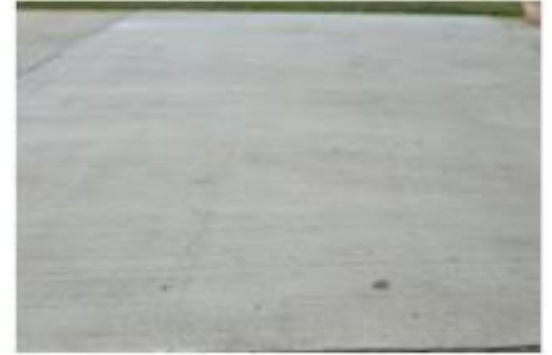
EdenCrete Trial Slab
