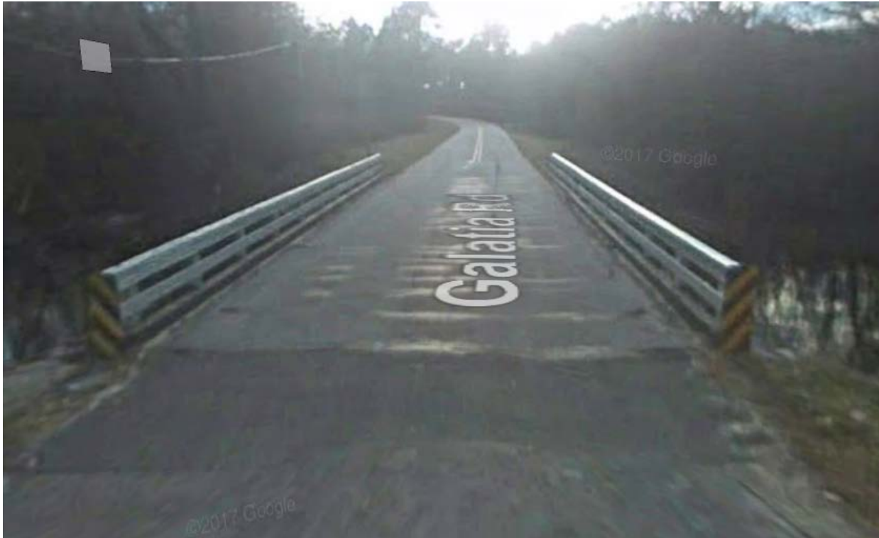
Figure 1. Bridge used for NCDOT trial
