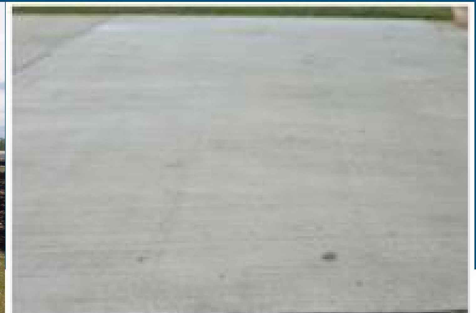
EdenCrete® TRIAL SLAB
