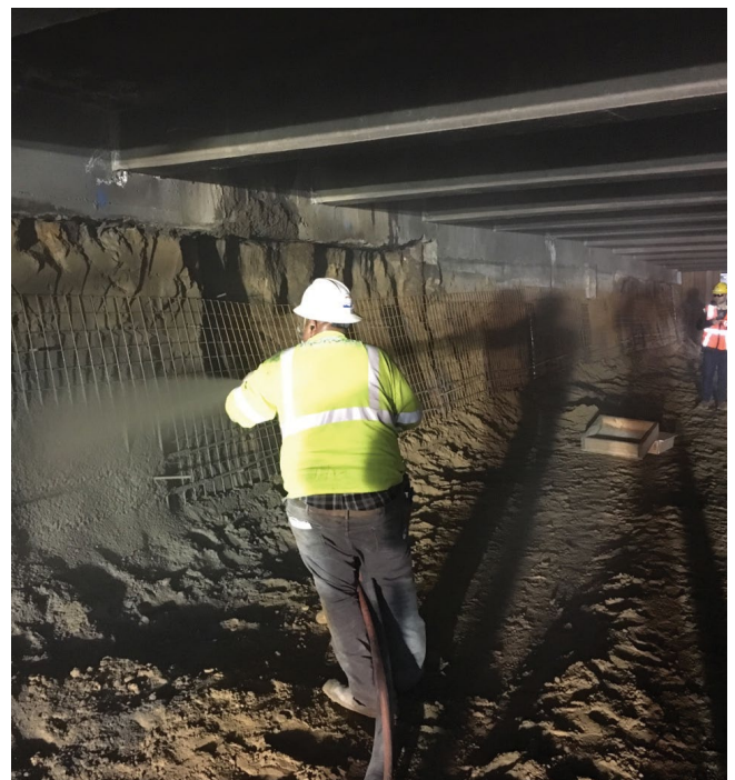
Figure 1. EdenCrete® shotcrete concrete mix being applied
