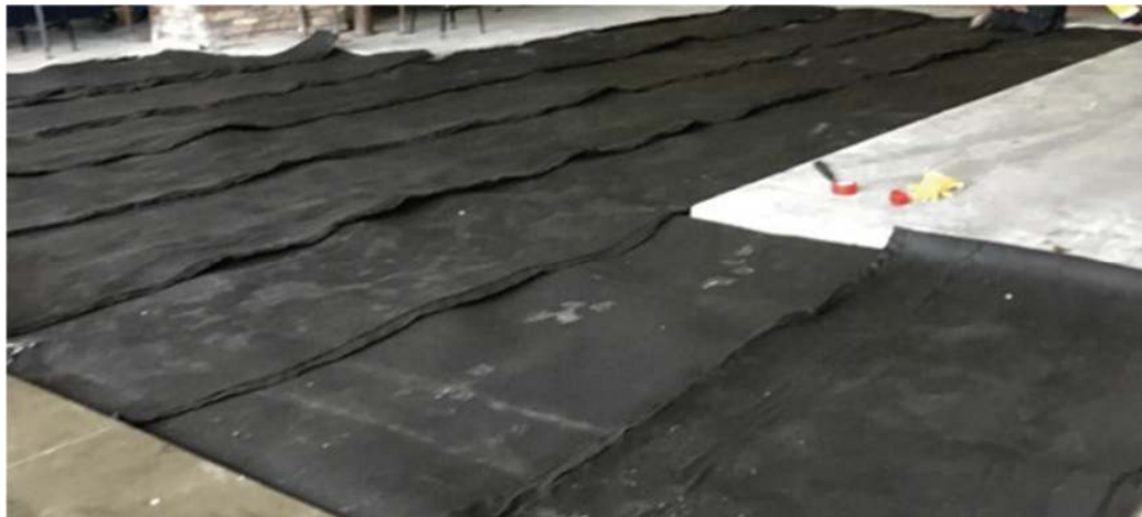
Figure 1. Interior Corridors- 3-inch-thick EdenCrete® concrete overlay on drainage system and suspended deck
