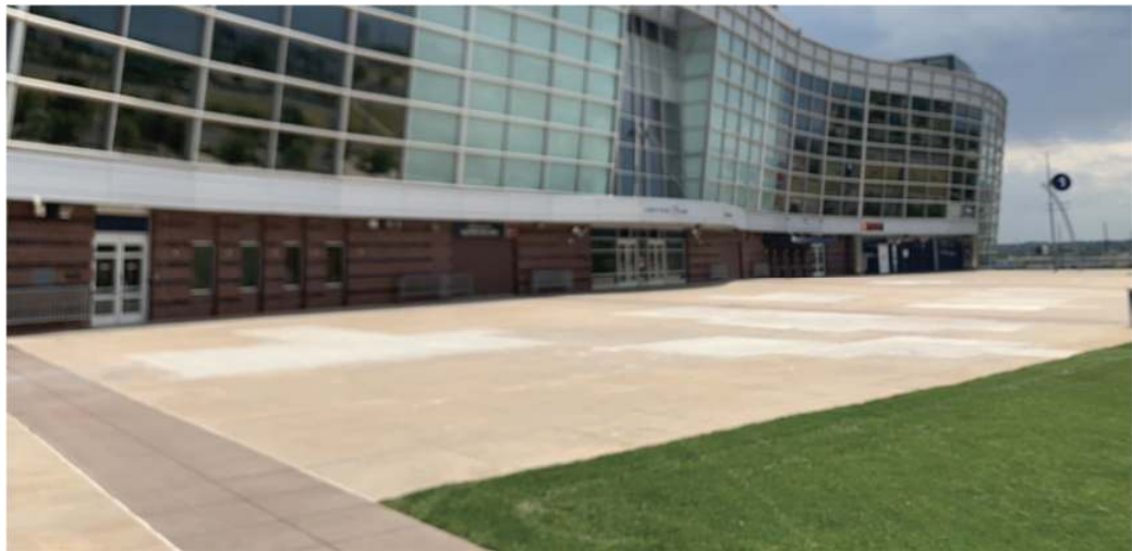
Figure 3. Exterior Corridors – 5-6-inch-thick full-depth slab
