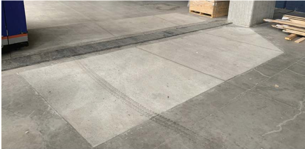
Figure 2. Interior Corridors- 4-inch-thick overlay on suspended slab
