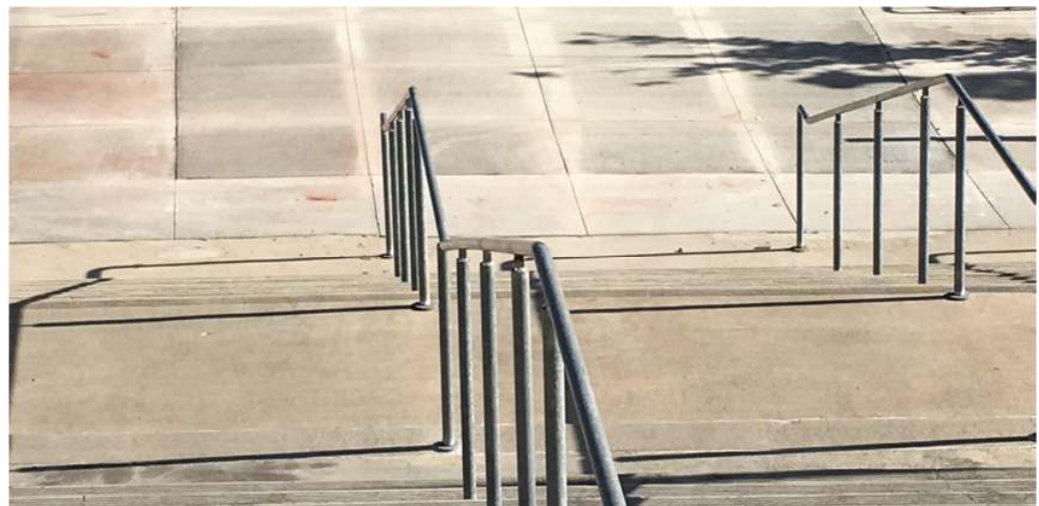
Figure 4. Perimeter Facilities - 5-6-inch-thick, full-depth slab repair.
