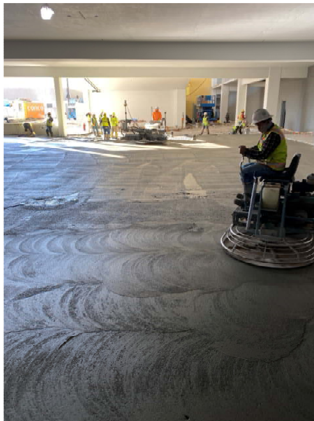
Figure 7. Slab on Grade being placed and finished
