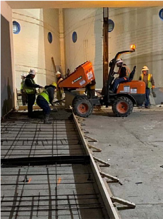
Figure 5. Interior sidewalk being installed
