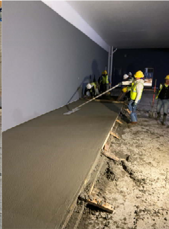
Figure 6. Interior sidewalk being finished
