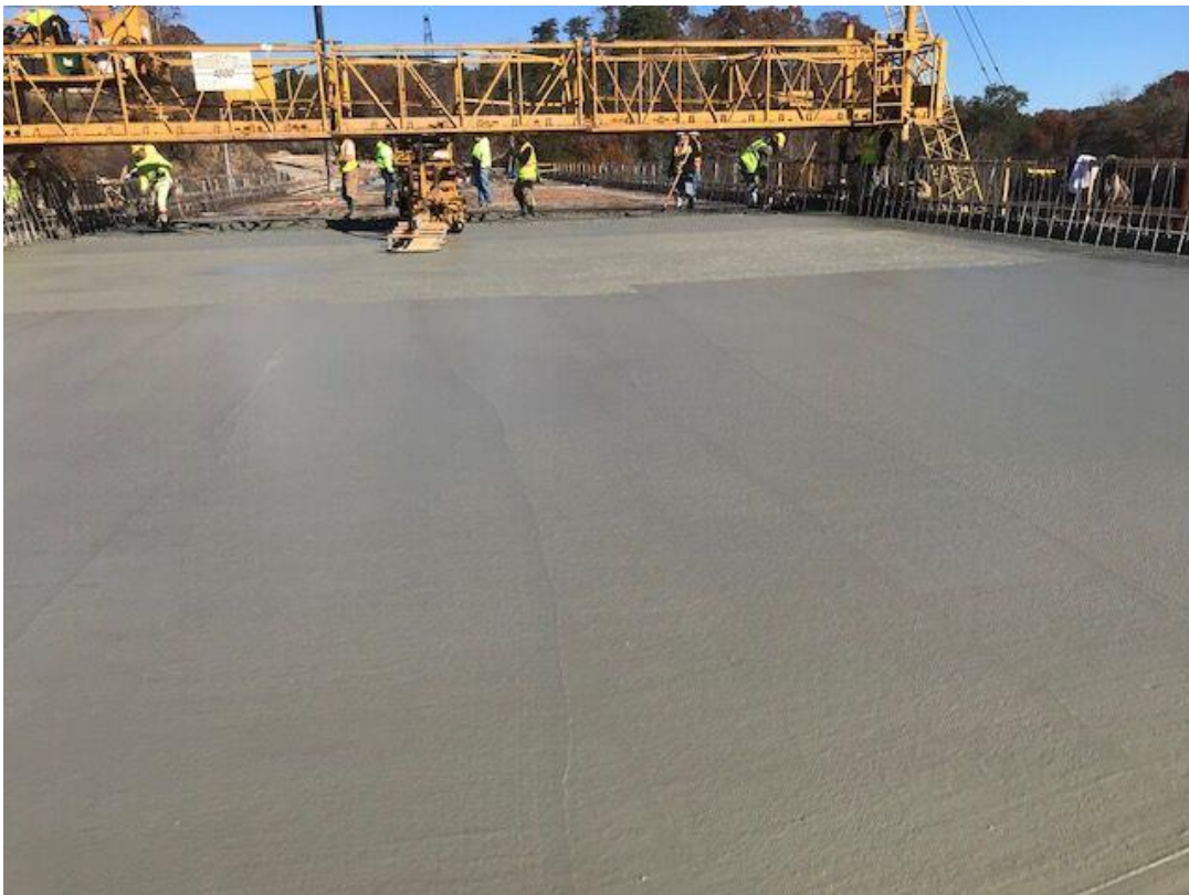
Figure 9. Little River bridge trial- showing freshly installed concrete in 2019
