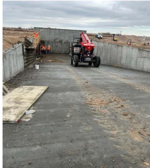
Figure 4. Longs Peak Dairy-fluid retention basin walls.
