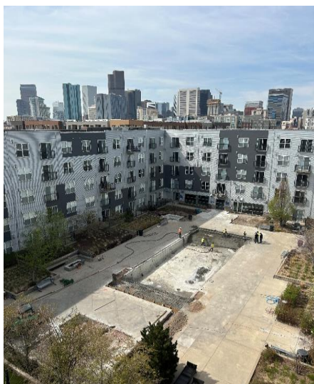
Figure 7. Ball Park Apartments, Denver.
