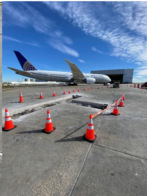
Figure 2. Concrete slabs being replaced
