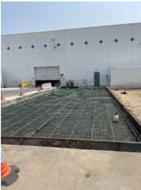
Figures 5 &6 DIA- United Cargo Area – concrete panel replacement.
