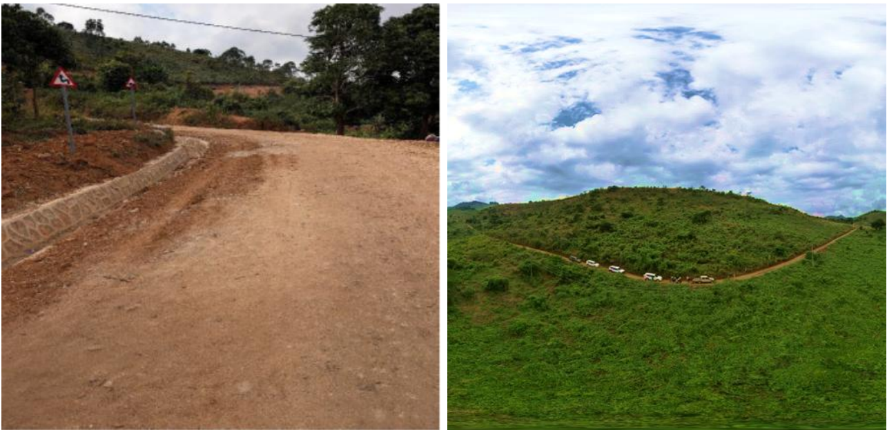
Figure 1 – Southern Access Road
