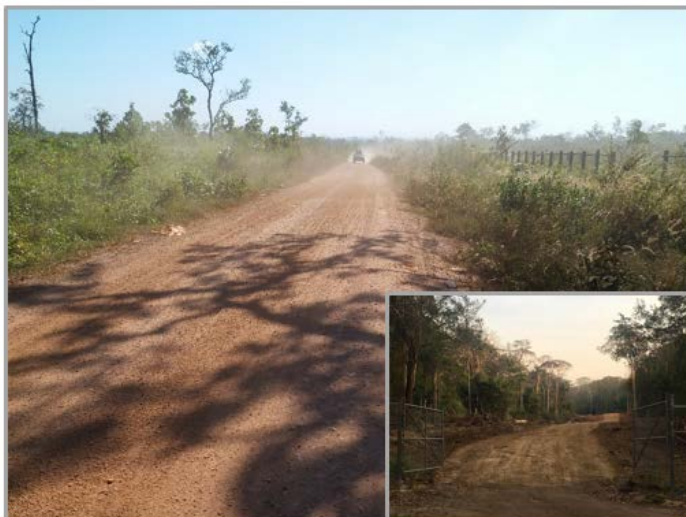
Figure 5 | New Road Construction
