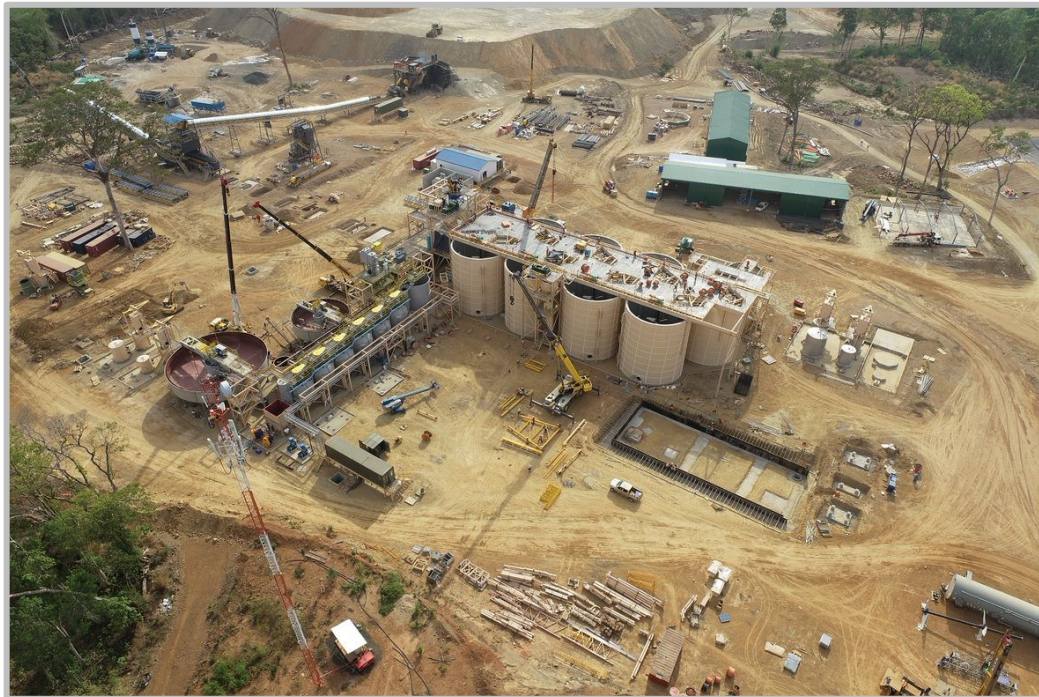
Figure 1 | Process Plant Progress - nearing completion
