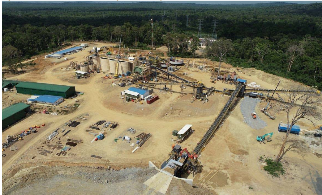
Figure 1 | Process Plant and Crushing Circuit - complete and commissioned
