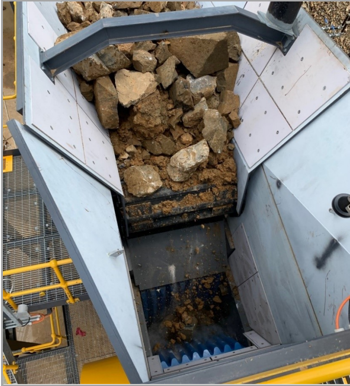
Figure 5 | Commissioning of the Jaw Crusher
