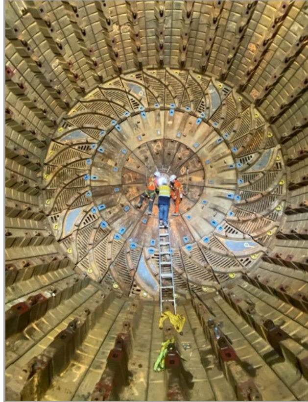
Figure 11 | Final mill liner segment installation
