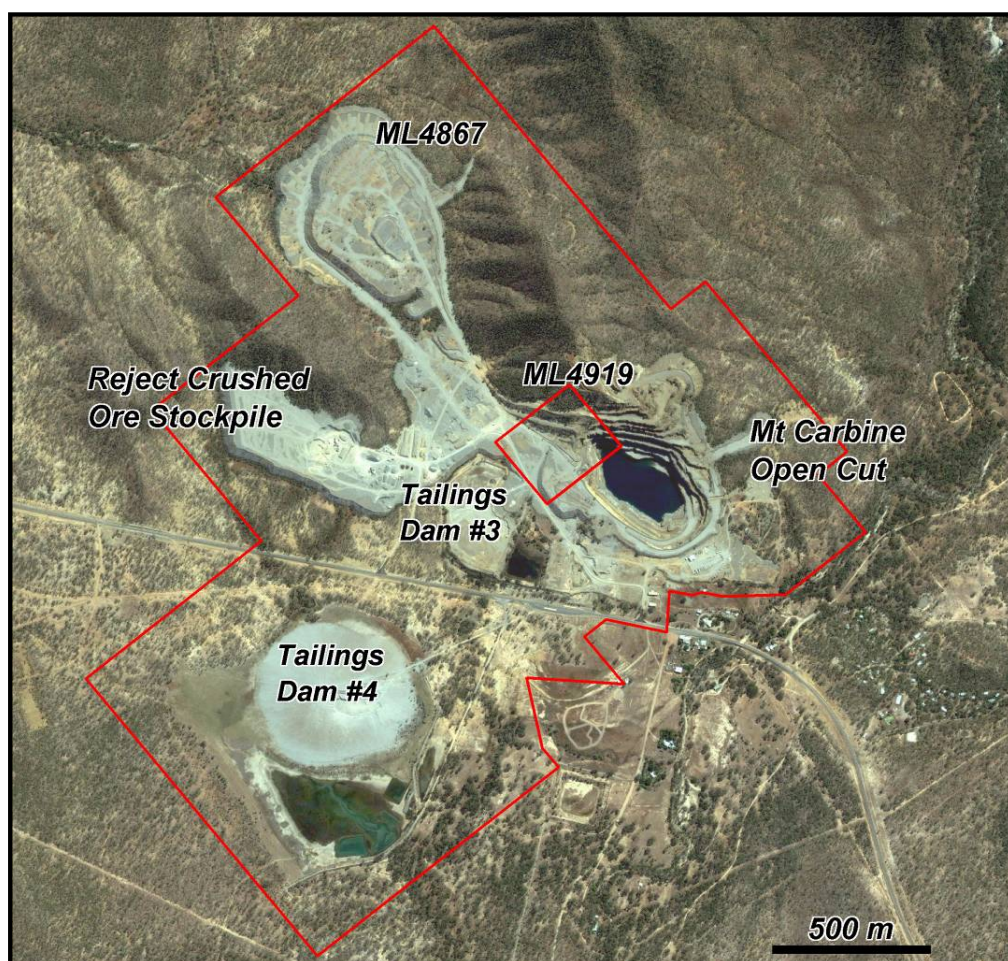
Mt Carbine Tungsten Project – Aerial View of Mining Leases showing the open cut, #3 and #4 tailings and waste dumps. Icon's strategy is to start by re-treating the tailings and, at the same time, prove up a viable primary ore resource in an expanded open cut.
