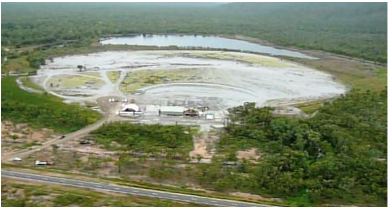
Aerial view of the tailings re-treatment plant, tailings stockpile and the water supply dam in the distance.
