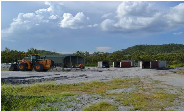
Office, stores and workshop area under construction at the right, shaker table shed at the left, Carbine Tungsten front-end loader in the foreground, low-grade stockpiles visible.
