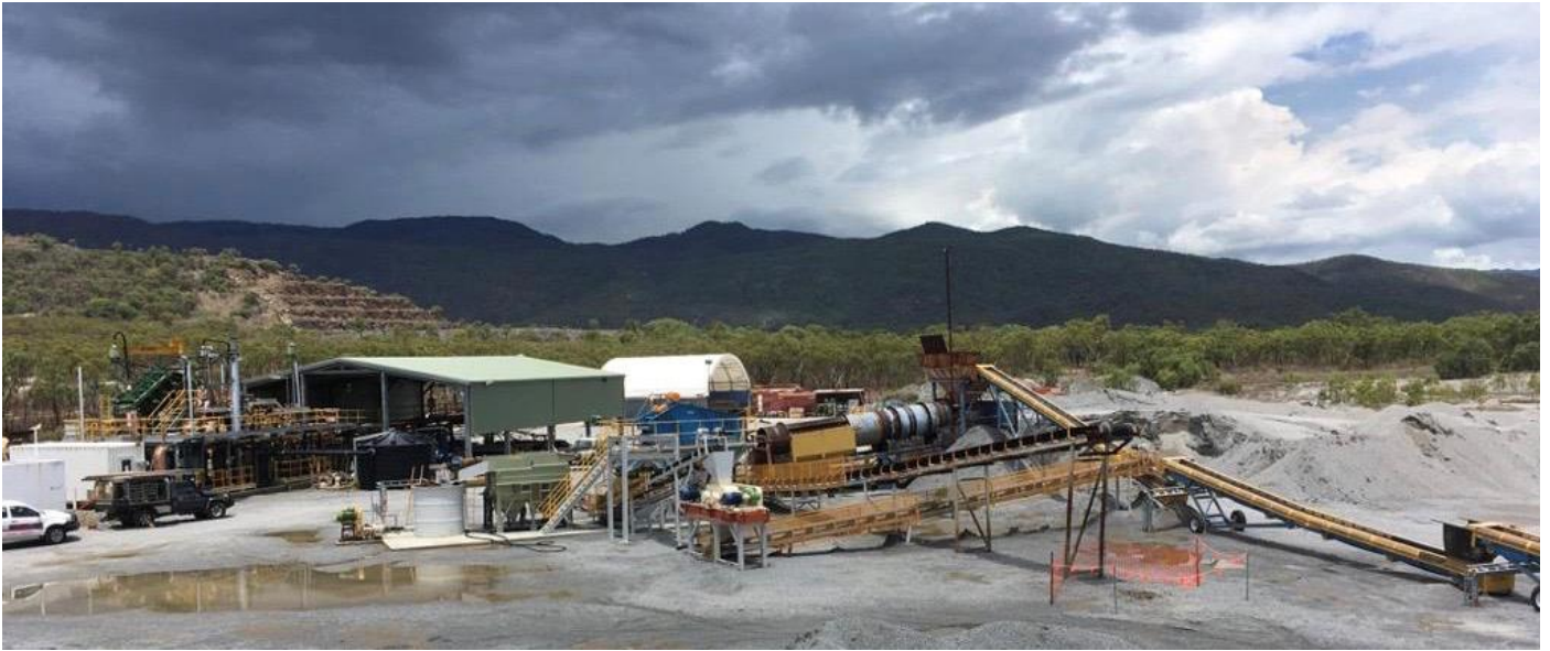
View of the commissioning of the Retreatment Plant (raw material intake at front right; screening, crushing and jigging at center front; gravity circuit under shed).
