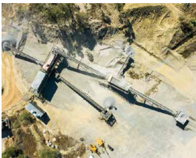
Aerial view of XRT Sorting plant
