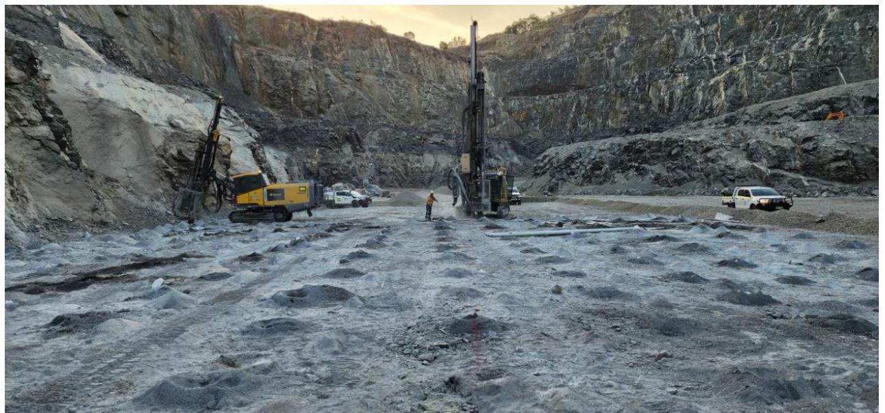
Figure 5: Orana Drill and Blast Rigs
