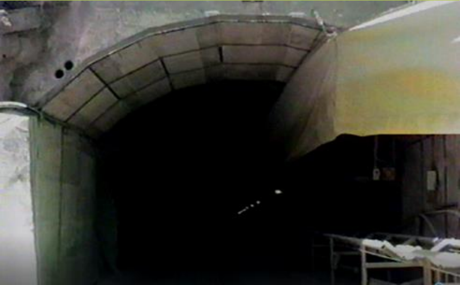
Mt Carbine Existing Decline - Historical Pictures 1986
