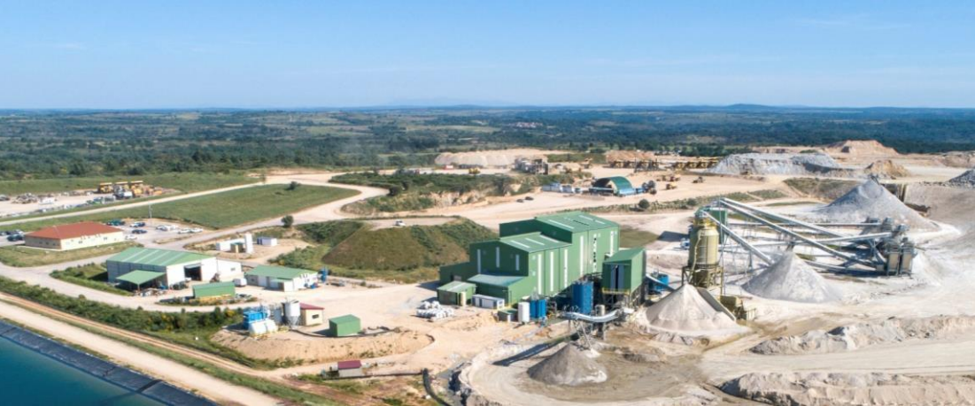
World-class Processing Plant
