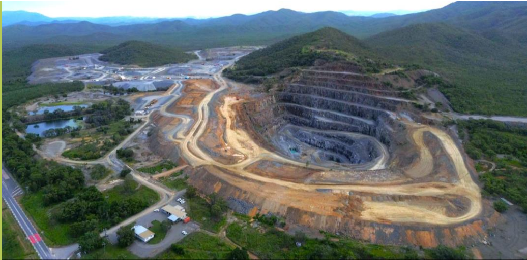
Mt Carbine Open Pit & Processing Plants
