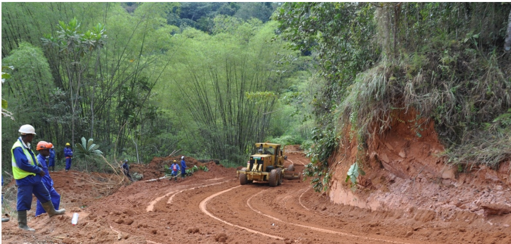
Figure 5: Deviation completed by Congo Mining for Leyou Bridge Refurbishment
