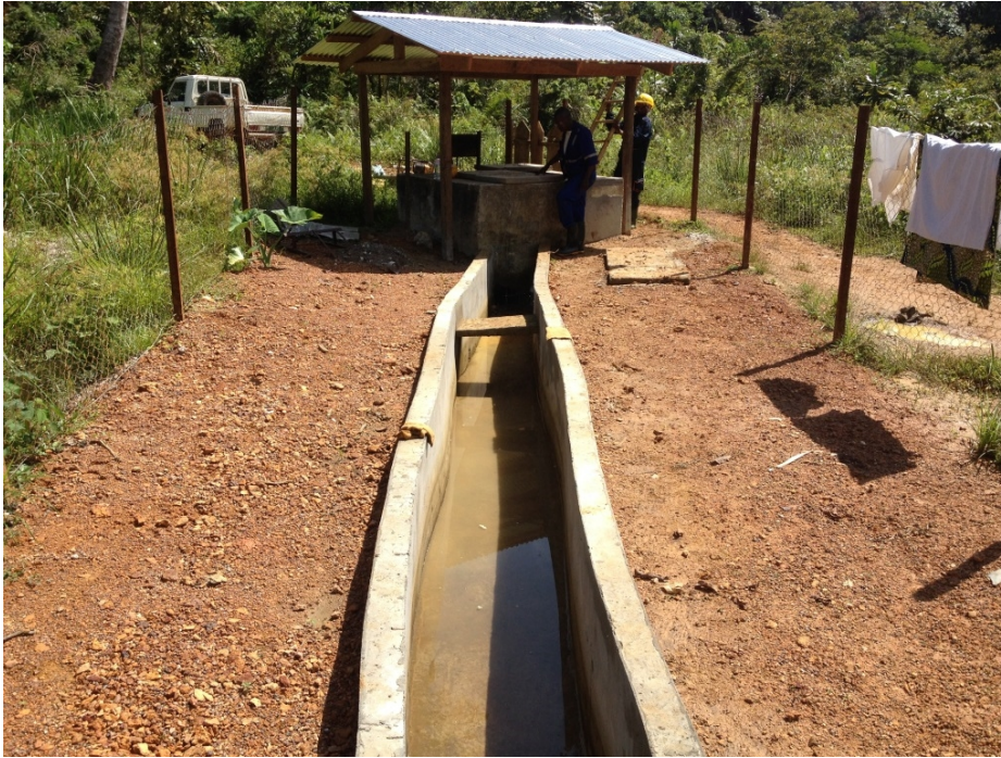
Figure 6: Maintenance on the Water Treatment Plant
