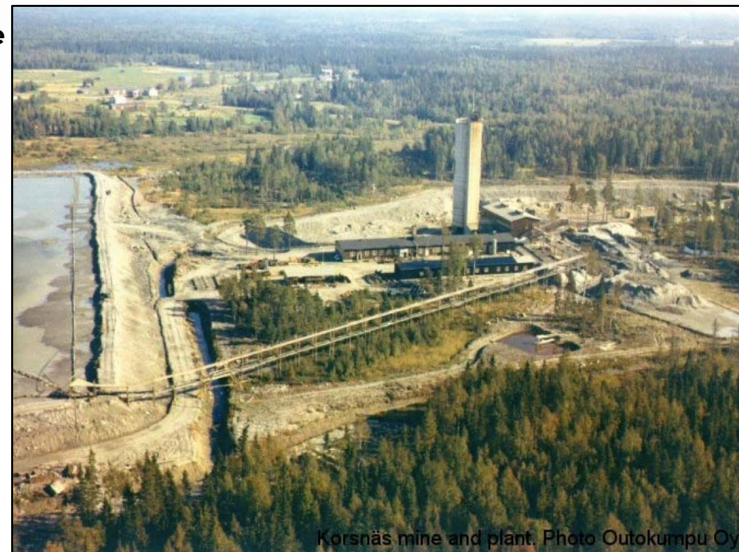
Korsnäs mine and plant. Photo Outokumpu Oy.
