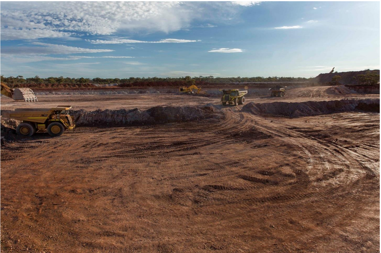
Penny's Find - digging in the hanging wall
