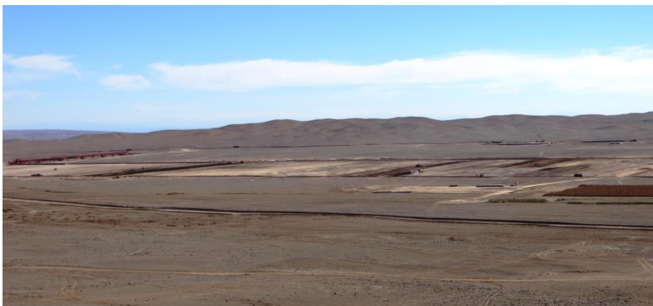
Figure 4: Photo taken by Estrella from Estrella's Antucoya West Prospect of Antofagasta Minerals' construction of heap-leach pads at their Antucoya mine development (January 2014).
