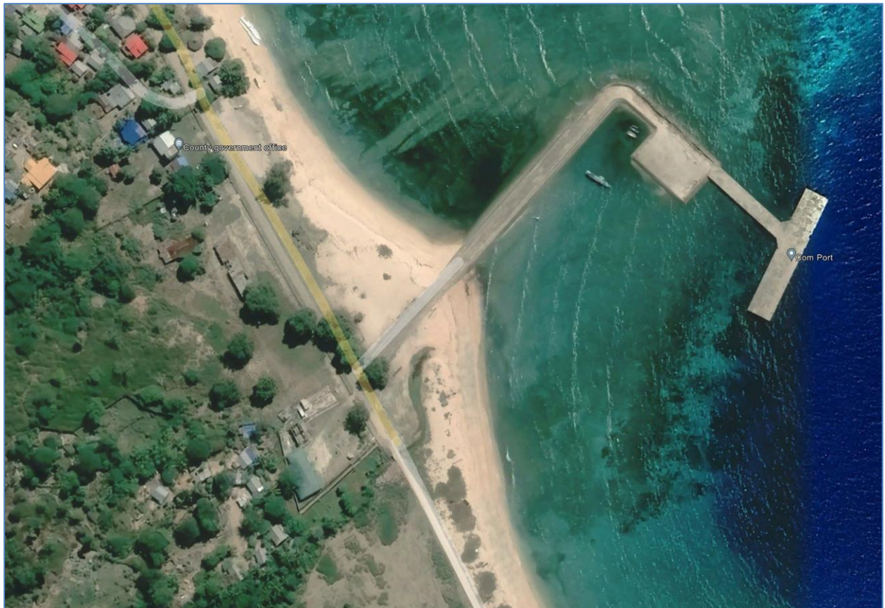
Figure 5: Aerial view of the Com deep-sea port
