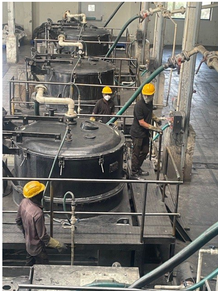
Figure 5 – Part of the Processing Plant final stage
