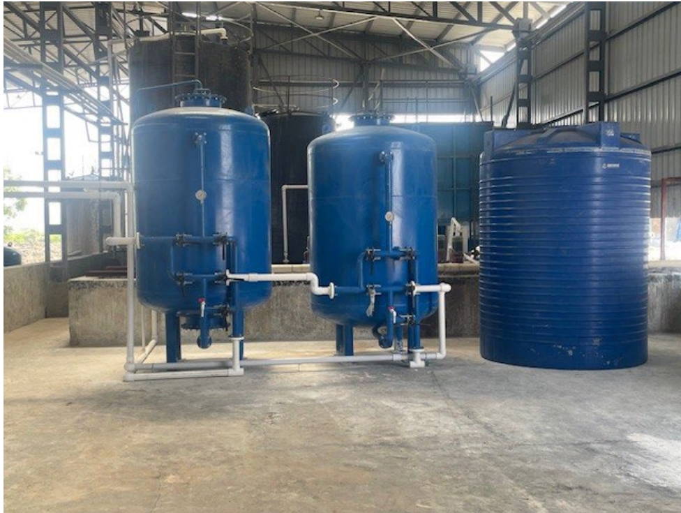
Figure 4 – Part of the effluent treatment plant that provides for 95% recycling of water
