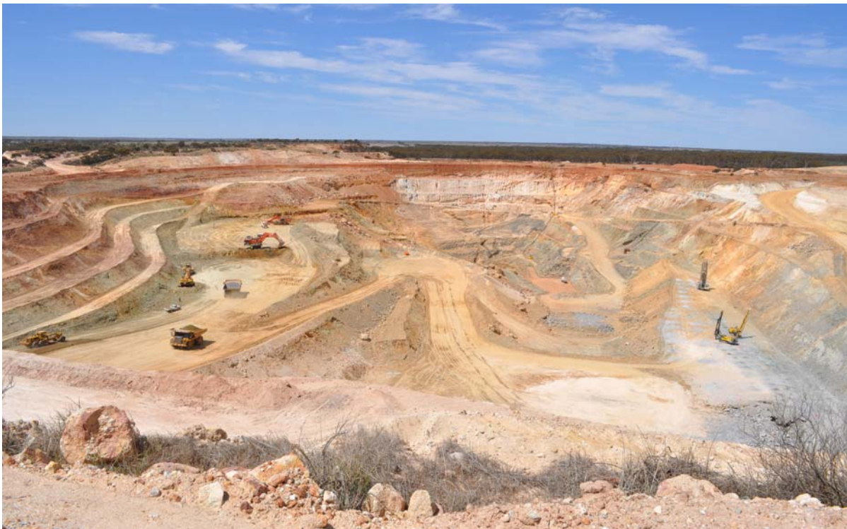
Figure 2 - View from the western end of the Edna May open pit showing the cutback of the failed upper oxide zone with flatten slopes ( LHS) and exposure fresh ore (bottom RHS).
