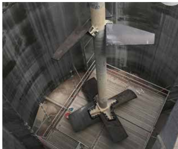
Looking inside one of the tanks
