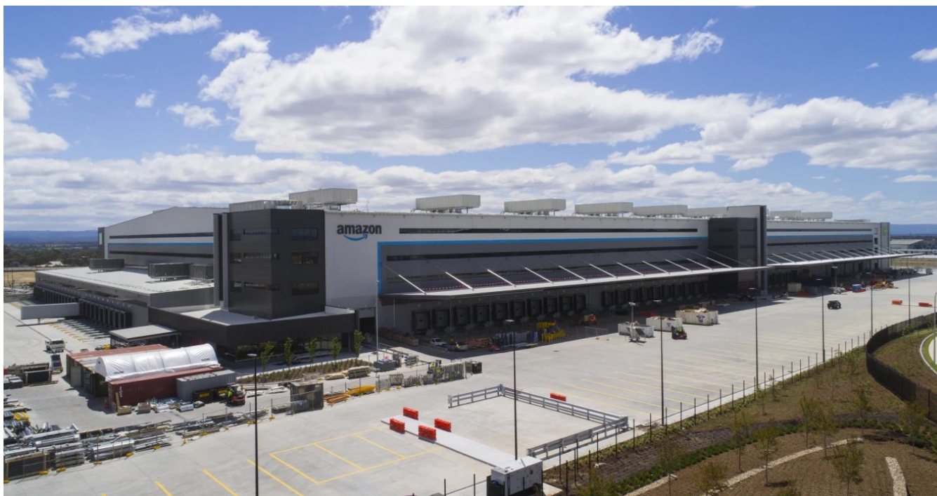
Amazon Robotic Fulfillment Centre – Syfon Systems project
