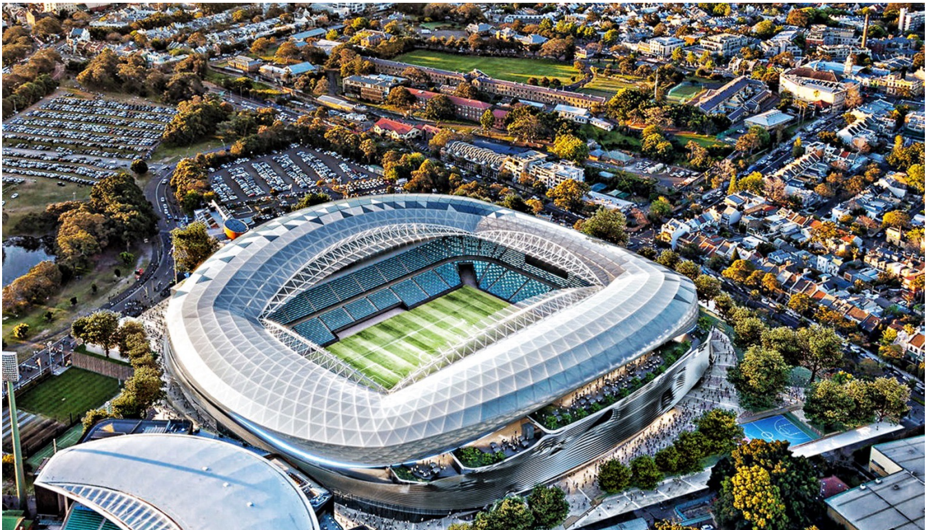
Sydney Football Stadium – Syfon Systems project underway
