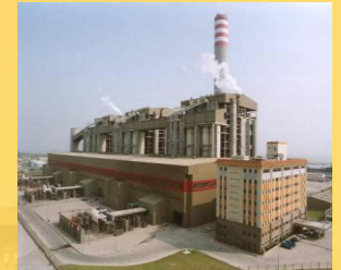
3 x 660 MW Shajiao C Power Plant, China
