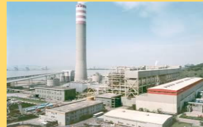
2 x 350 MW Shajiao B Power Plant, China
