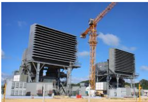
Construction of Power Plant
