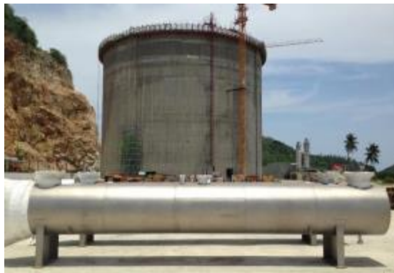
Installation of Regasification Unit
