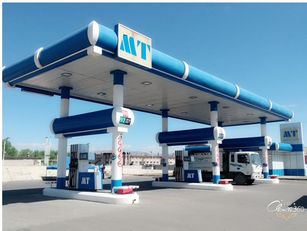
A MT Group Service Station
