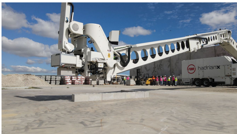
Next-generation Hadrian X ® commences first outdoor test build and live demonstration
