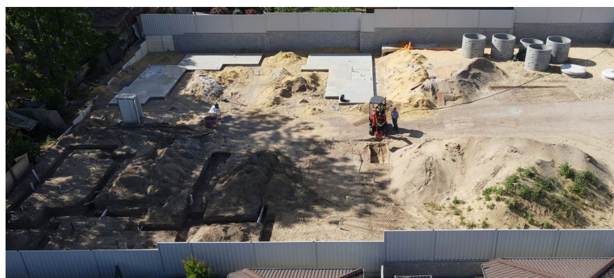
St. James – Early works and slab pouring under way
