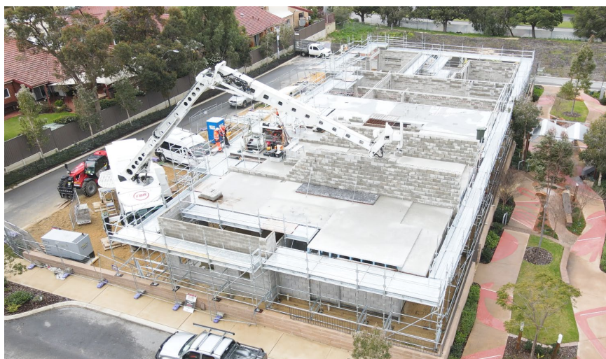
H02 constructing the second storey walls at Willagee
