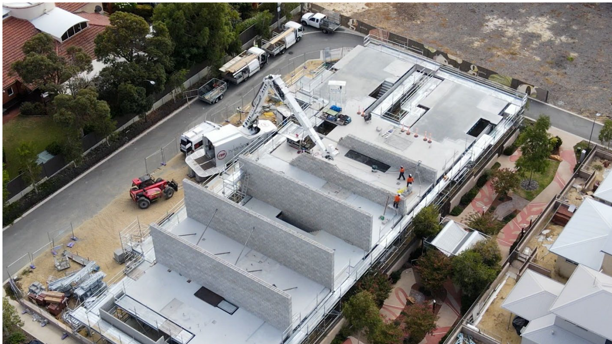
H02 completing the second storey common-party walls of the final stage at Willagee
