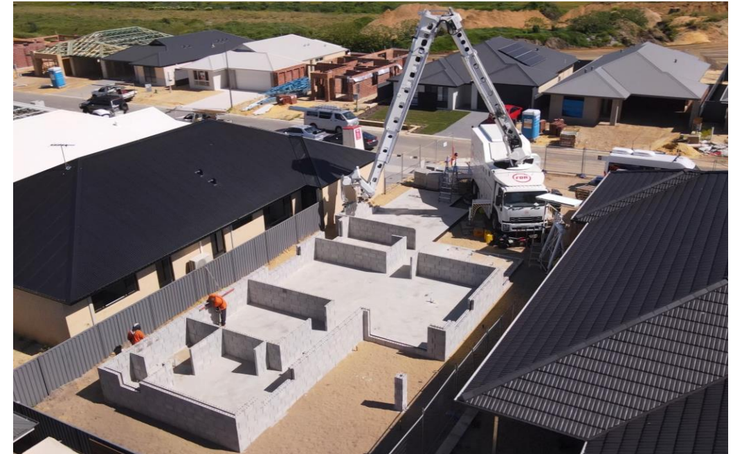
Hadrian X® building a structure in Perth, generating zero on-site masonry waste
