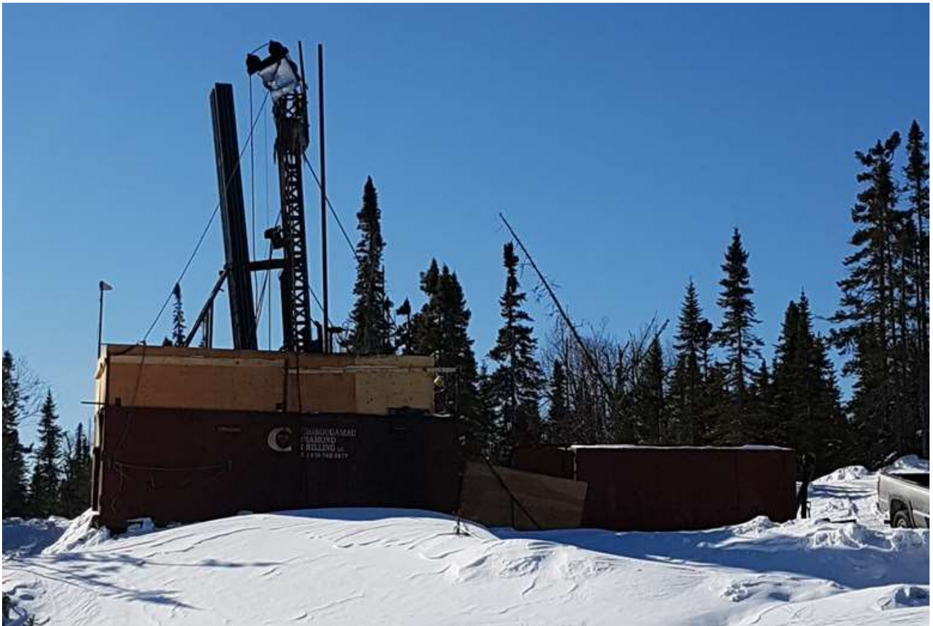
Image 2: Drilling at Pick Lake
