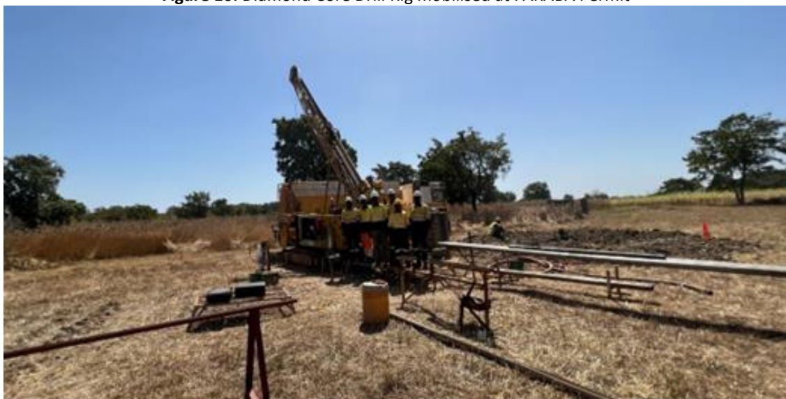
Figure 10: Diamond Core Drill Rig mobilised at FARABA Permit
