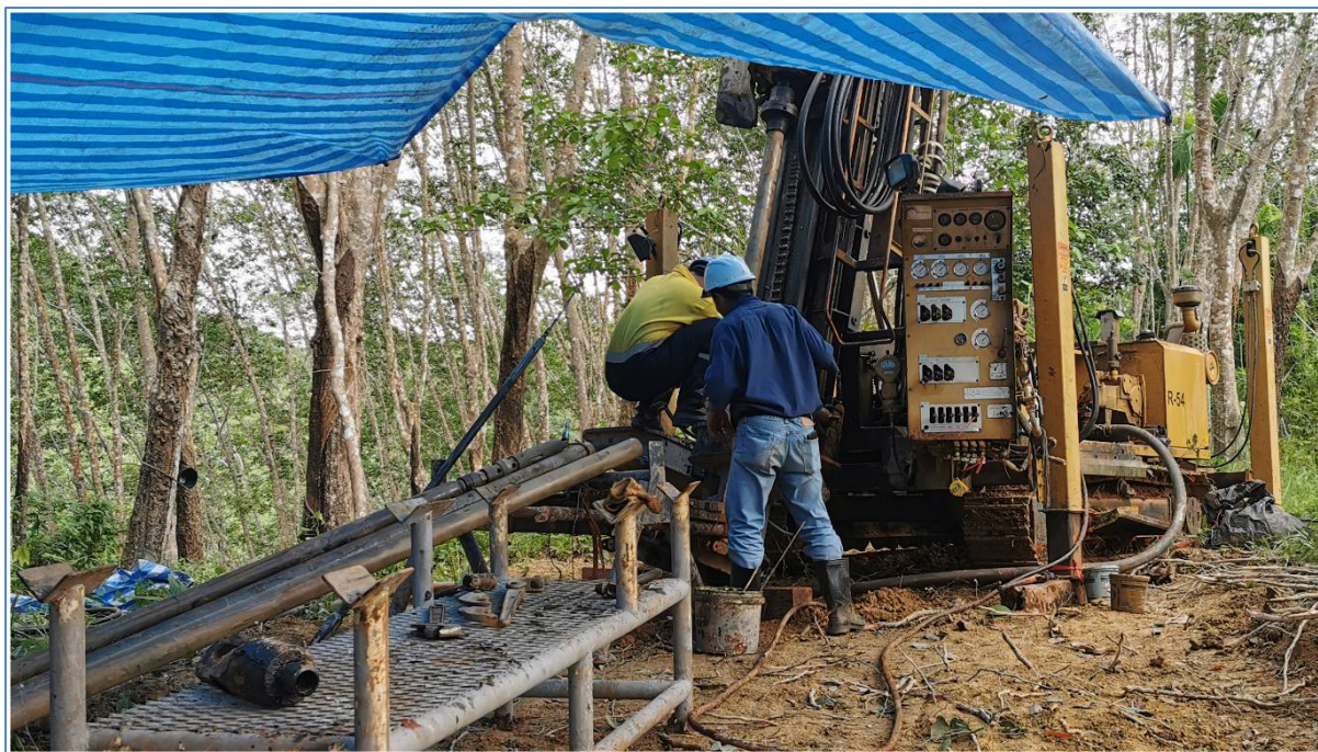
Picture 1: Khao Soon Tungsten Project – DrillCorp setting up for KSDD026, drilling with HQ diameter rods
