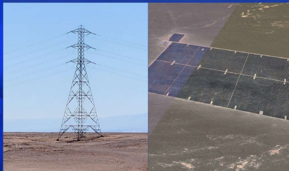
Substantial Energy Infrastructure
