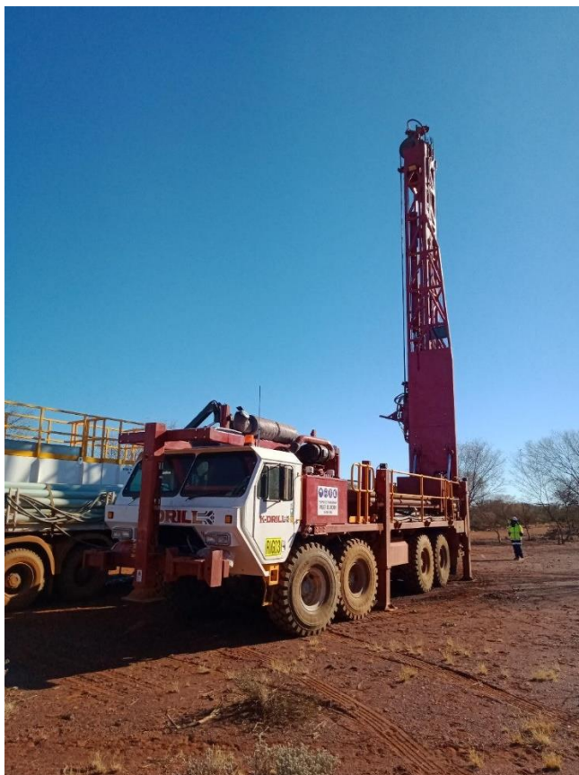
K Drill rig arriving on Site
