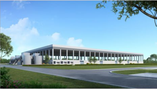
Ore & Tailing Storage, Calcining Kiln
