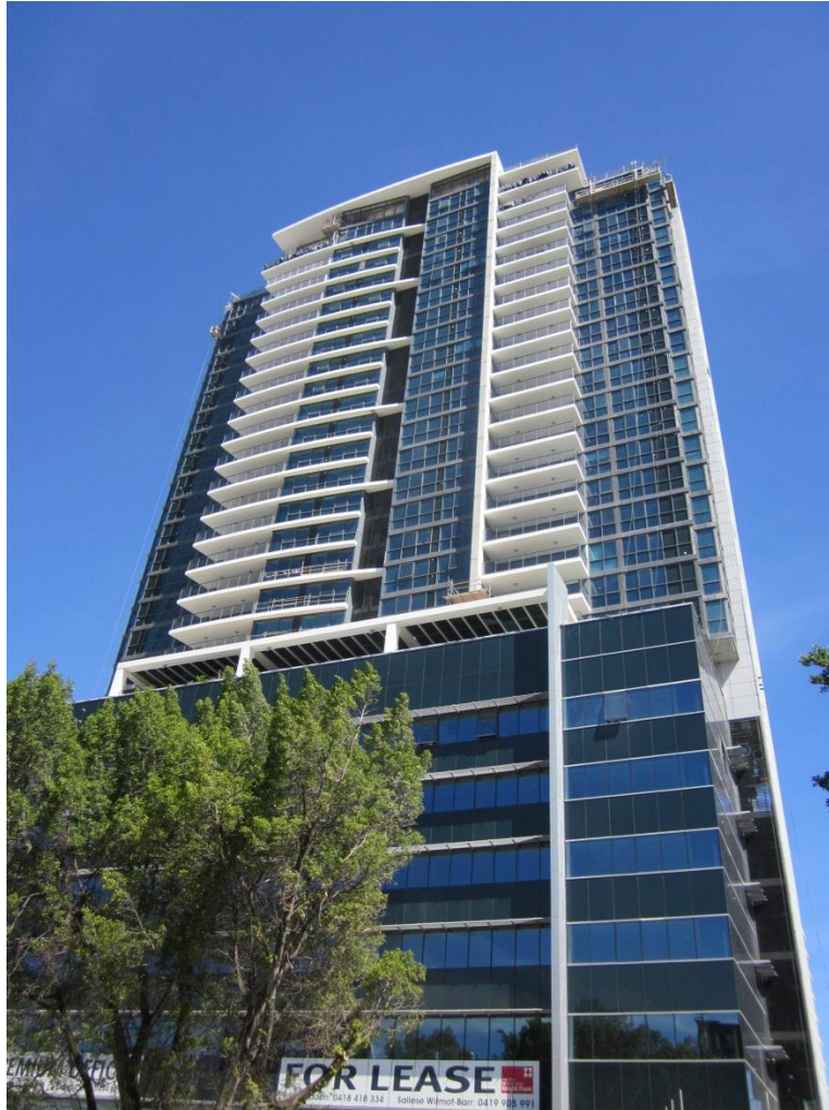
Photograph: Fairlanes, Practical Completion.
