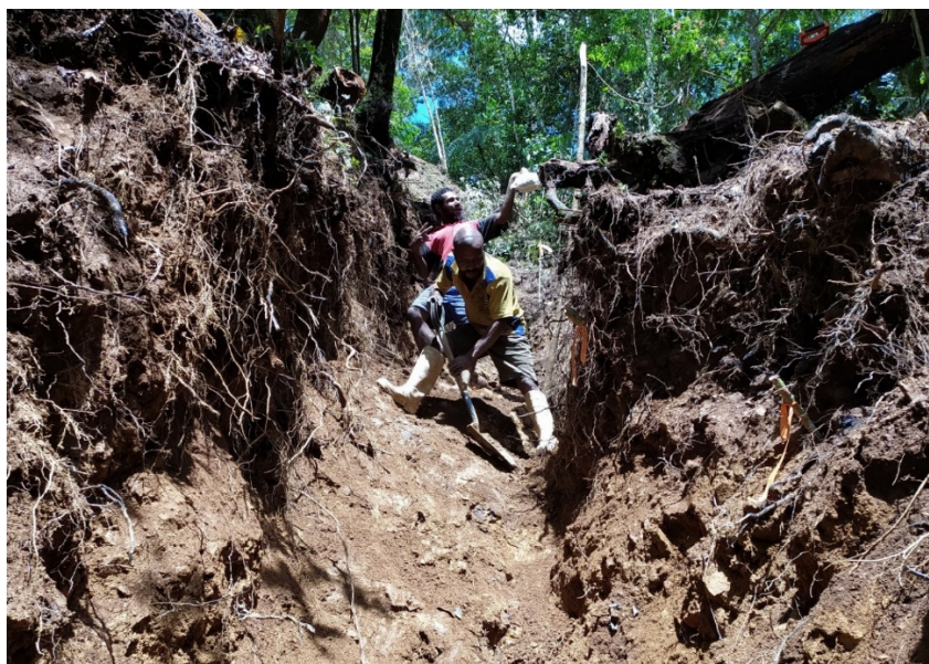
Photo 1: Digging Out Trench KC24 Before Sampling
